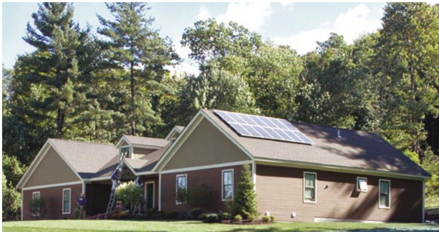
The Vitale's ICF home after the makeover.
