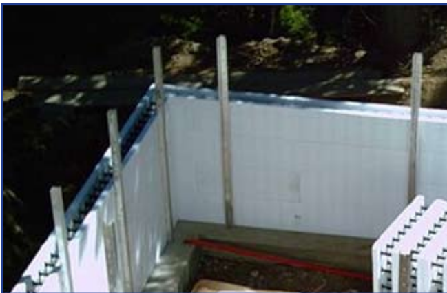
Minimal Inner Bracing
